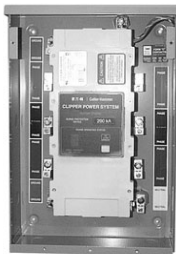
Interior View of a Retrofit Visor
